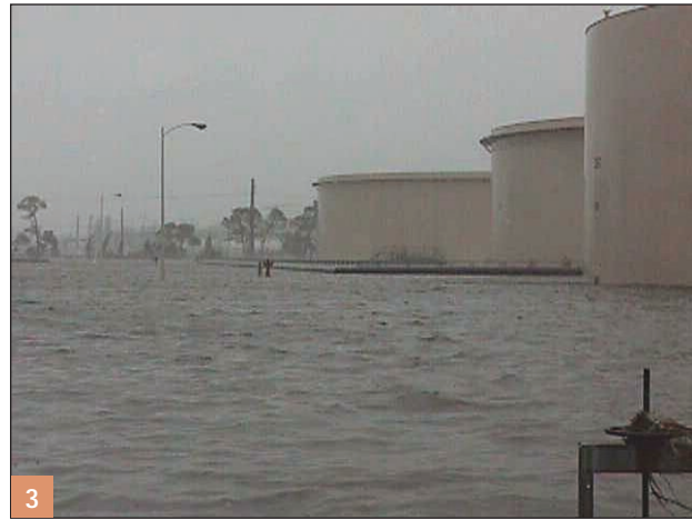
The 12-ft storm surge quickly overcame the refinery's 9-ft levies, flooding the facility in up to 5 ft of seawater in the office building, units, and tank farm alike.
