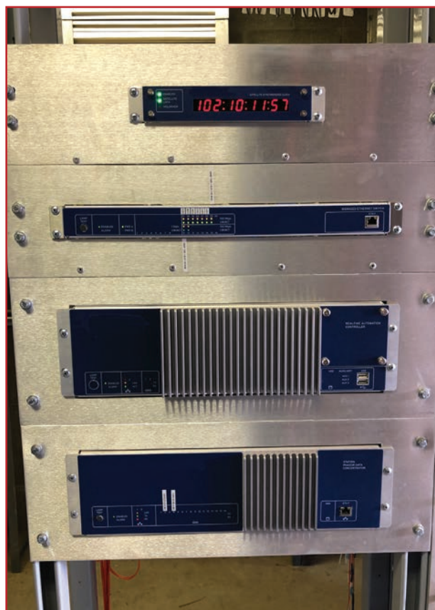
figure 6. The FCP substation IEDs. (Source: SDG&E.)
